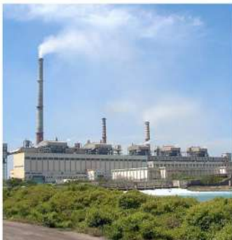
Bharat Heavy Electricals Ltd-Bhopal
